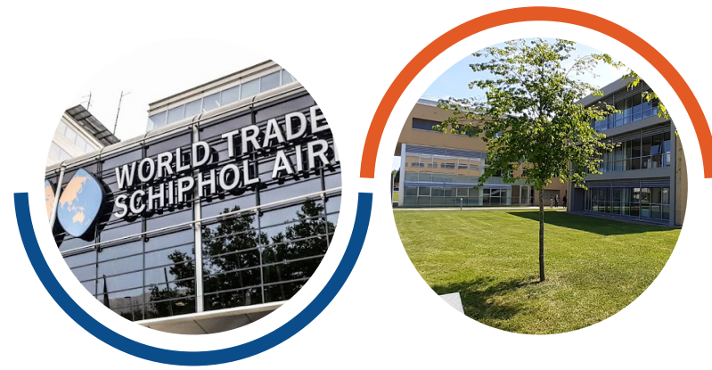
Operating WTC Schiphol Airport
